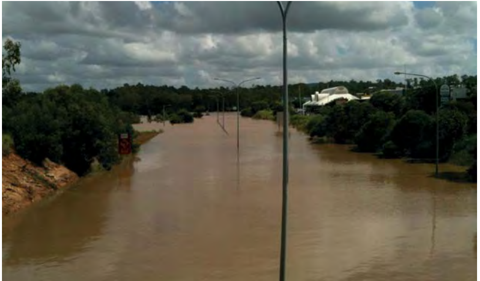
Jindalee overpass looking toward Centenary Bridge.
